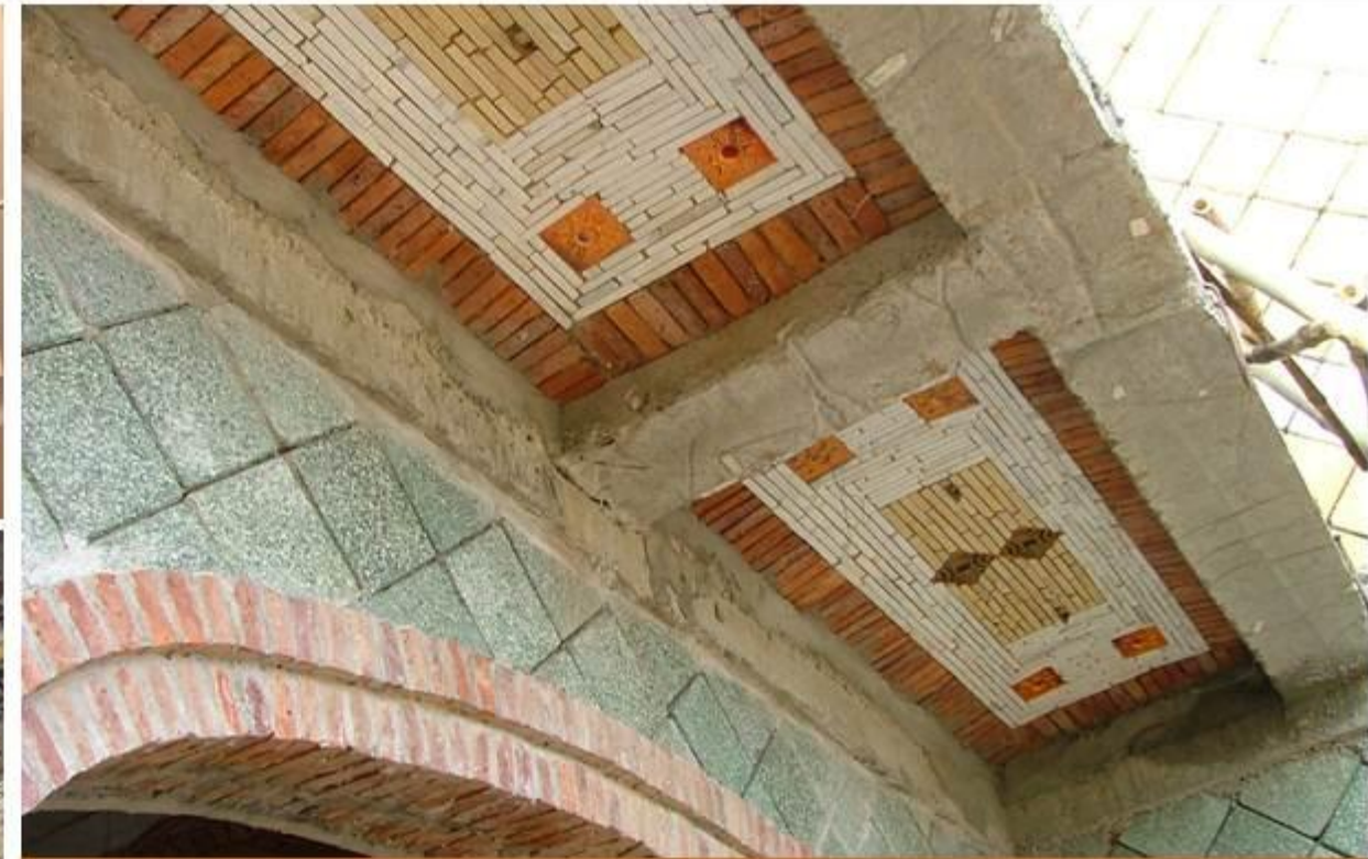
ROOFING SYSTEM - FUNICULAR SHELLS - using no steel in the shells MADE OUT OF RECYCLED MATERIAL
