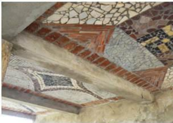
ROOFING SYSTEM - FUNICULAR SHELLS - using no steel in the shells MADE OUT OF RECYCLED MATERIAL
